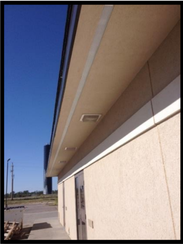
Repaired Soffit which was deteriorating. 2013.
